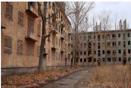
Figure 1: Abandoned panel houses, Kurchatov City
