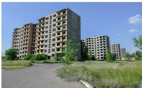
Figure 3: Abandoned panel houses, RTI micro-district, Saran (Turar Kazangapov)
