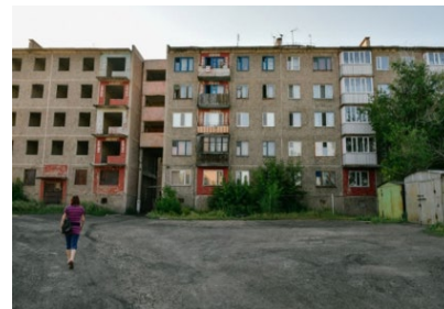
Figure 2: Abandoned panel houses, RTI micro-district, Saran (Turar Kazangapov)
